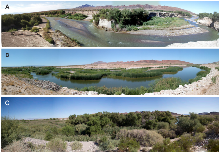
FIGURE 17. Calico Ridge Weir impoundment at the Las Vegas Wash: (A) 2000, pre-weir construction, showing tamarisk perched on tall terrace; (B) 2005, following weir completion and initial revegetation; (C) 2017, mature.
